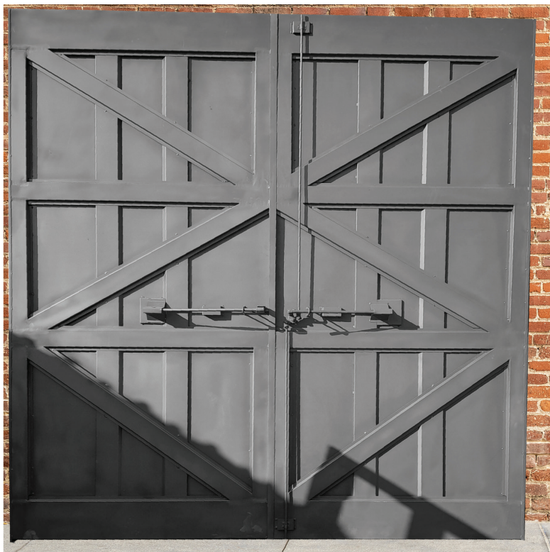
Oversize Door with Extra Bracing 3000 x 3000
